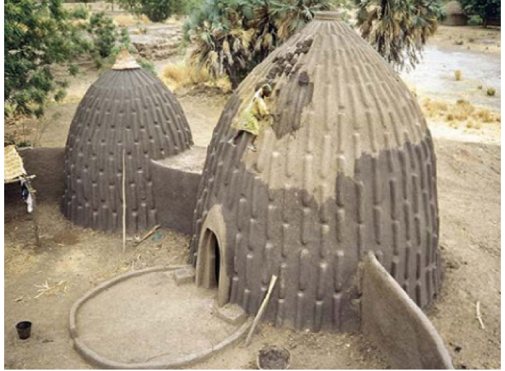
Stabilized Raw Earth Construction using Dung and Manure (Nubian Arch)
